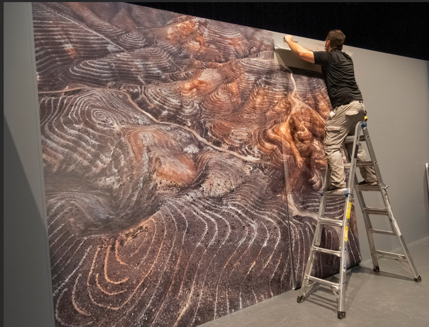
Wallcovering Install at The Canadian Opera Club
